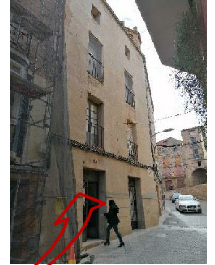
JUNCOSA Old Town Hall building
