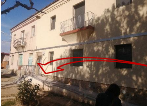
GRANADELLA Old building housing the teachers
